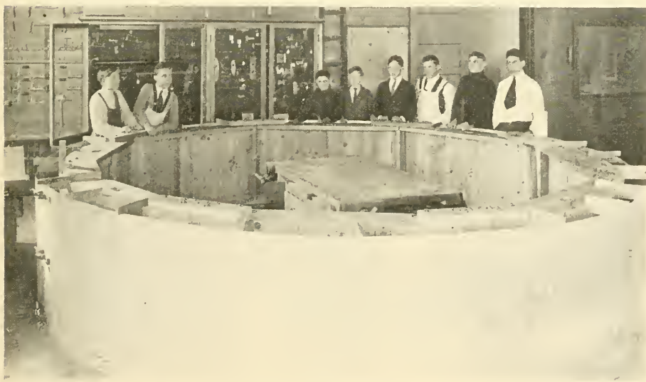
Fig. 41. Silo Form Completed.
